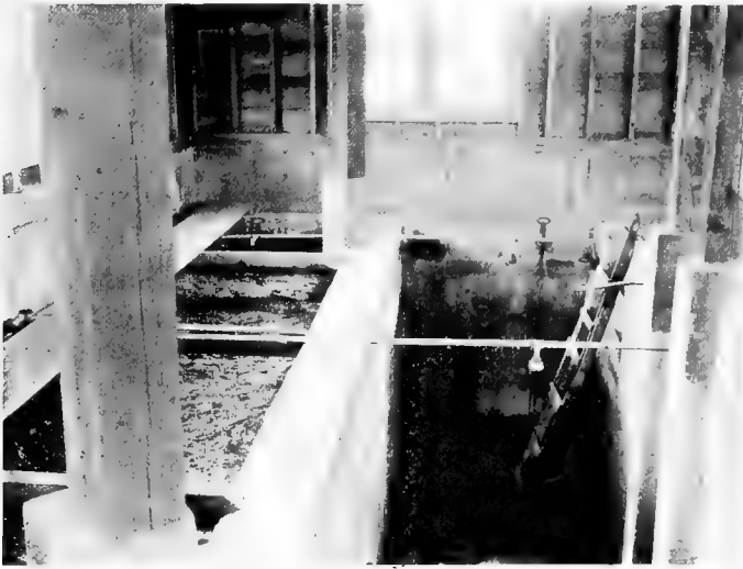
Fig. 43.—Two settling tanks—one empty and one filled.
